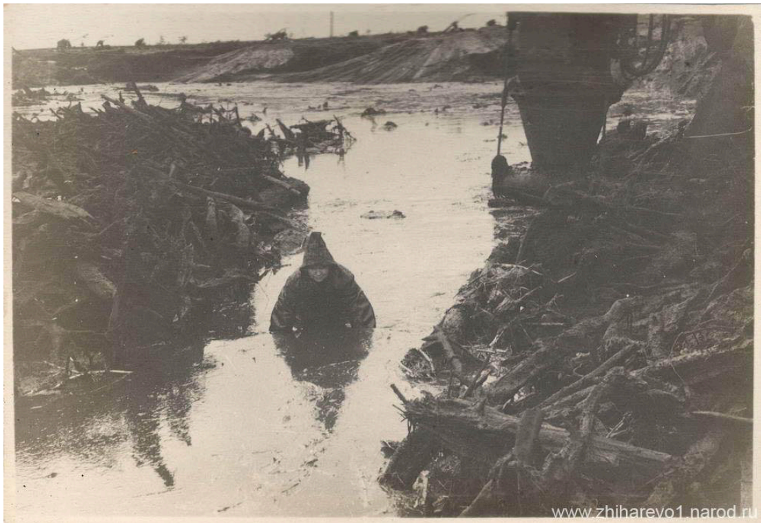
Pic. 4. Female peat worker in the peat liquid, pushing snags away to keep them out of the pipe. Leningrad Oblast, circa 1930-35. Author unknown.
